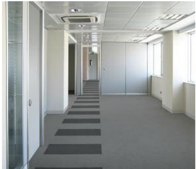
Consulco_Nicosia_Cyprus fully steel encapsulated panel calcium sulphate 30,5 mm › top covering: carpet lay-loose tiles
